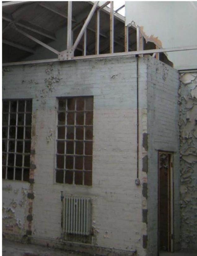
Fig 27: Existing radiators such as this one in Building 90, will be re-used if possible
